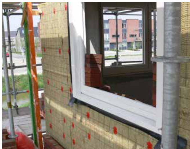
Prikspouwanker met UNI-CLIP
